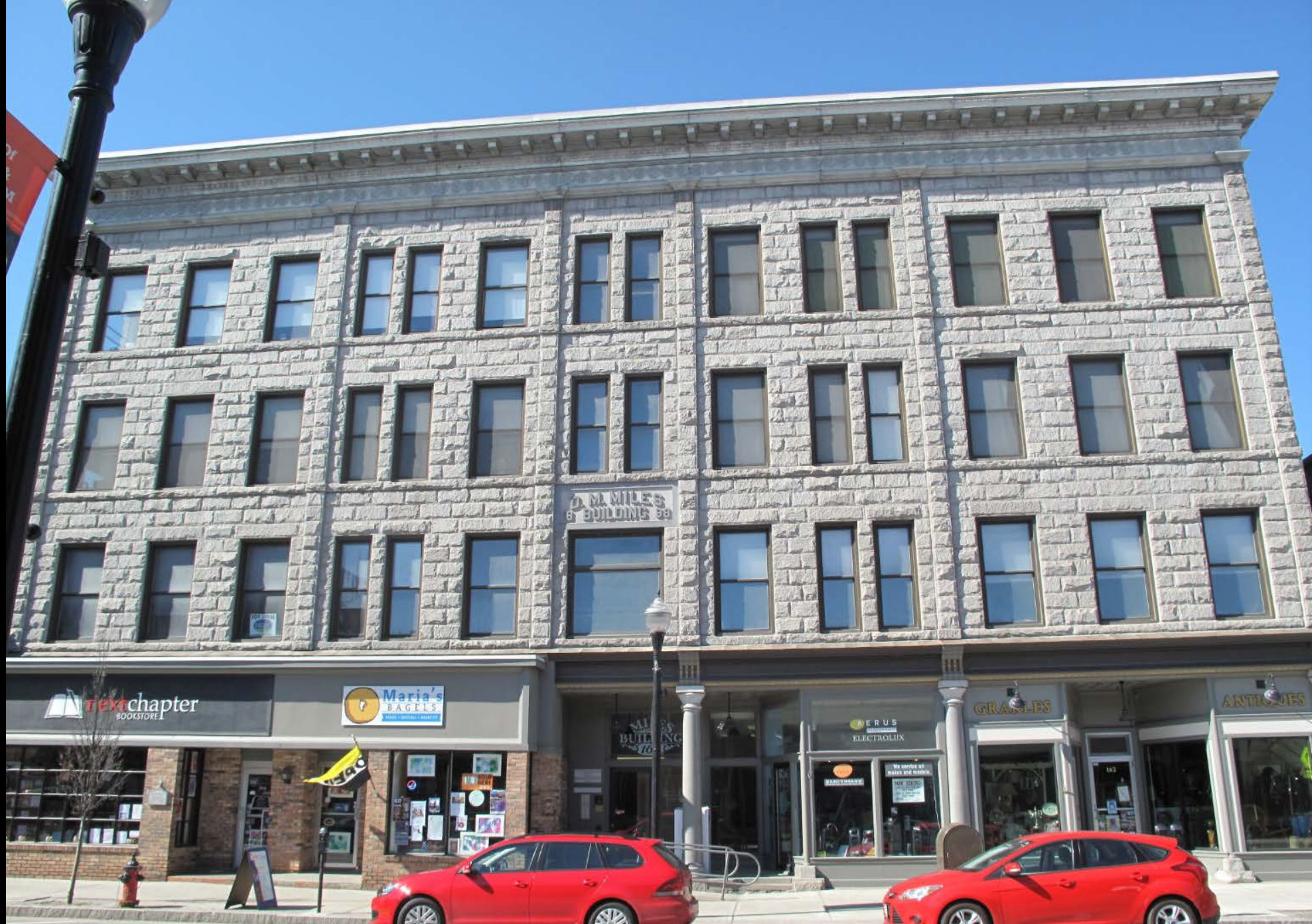
Photograph 42: View looking southwest at D.M. Miles Building, HD #27
