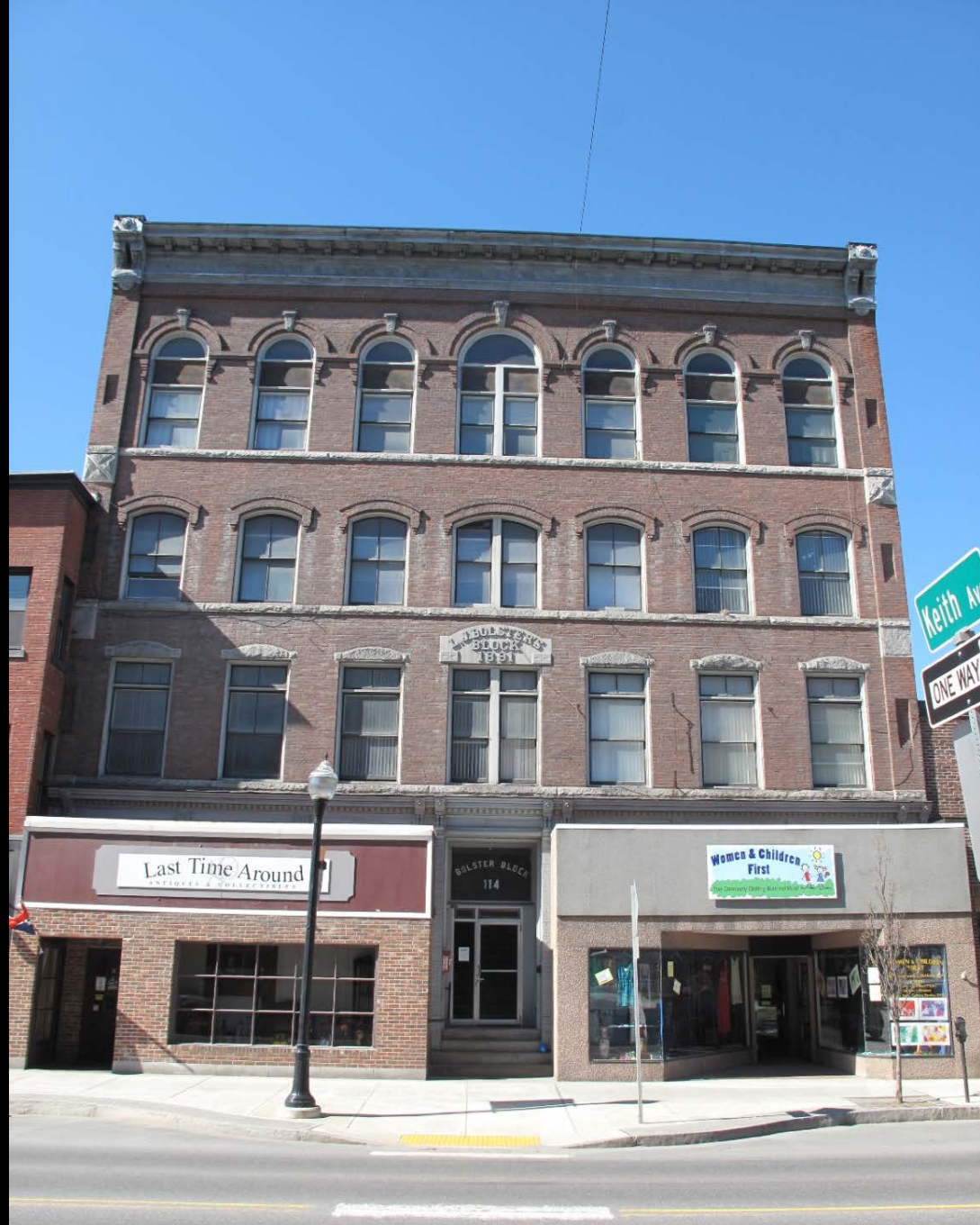
Photograph 40: View looking southwest at L.J. Bolster Block, HD #24
