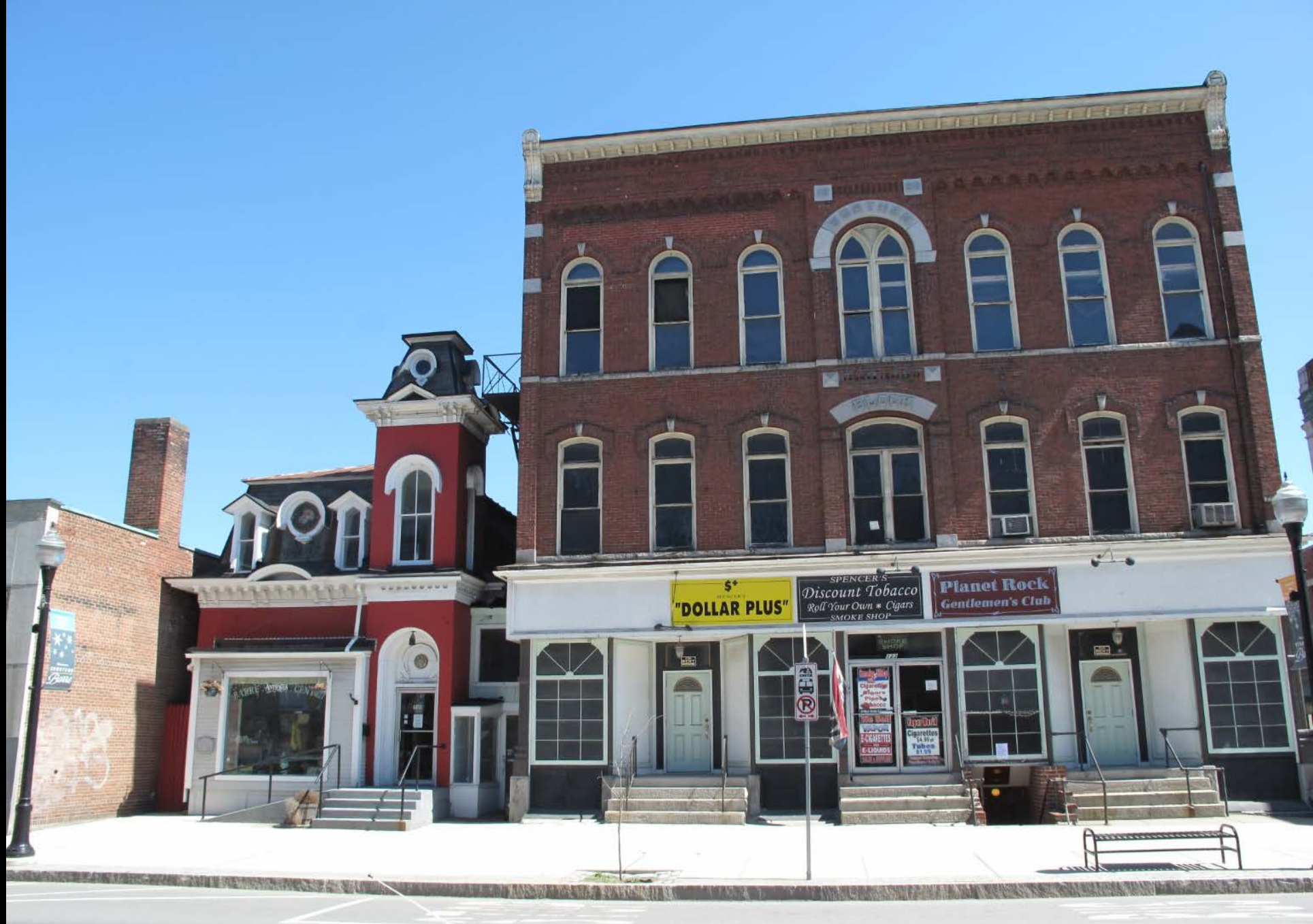
Photograph 57: View looking northeast at Wheelock Law Office (left), HD #42, and Worthen Block (right), HD #43
