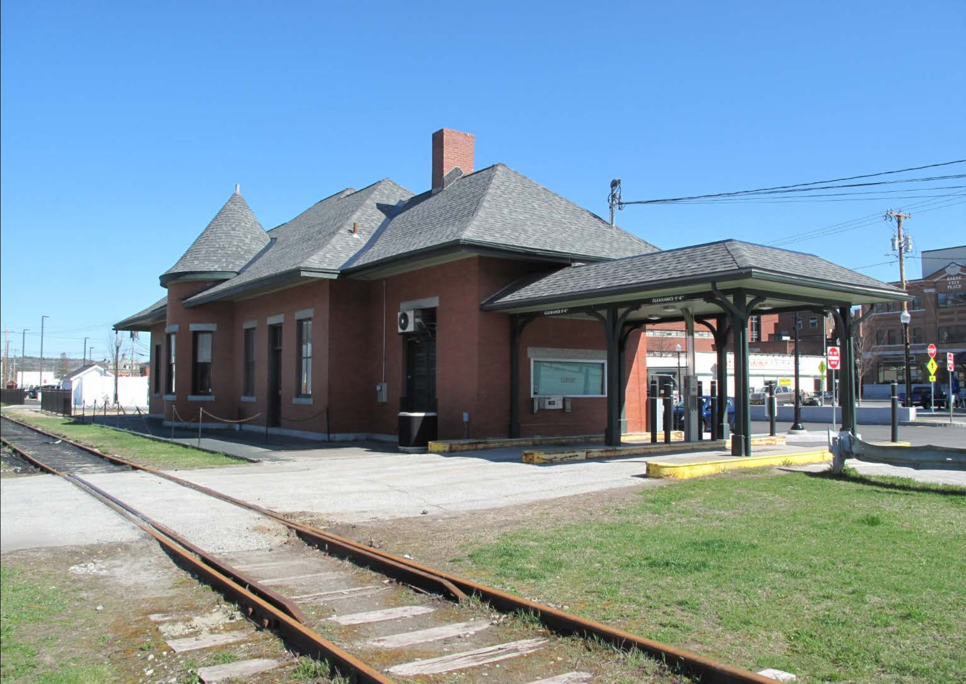
Photograph 49: View looking north at Vermont Central Passenger Depot, HD #35
