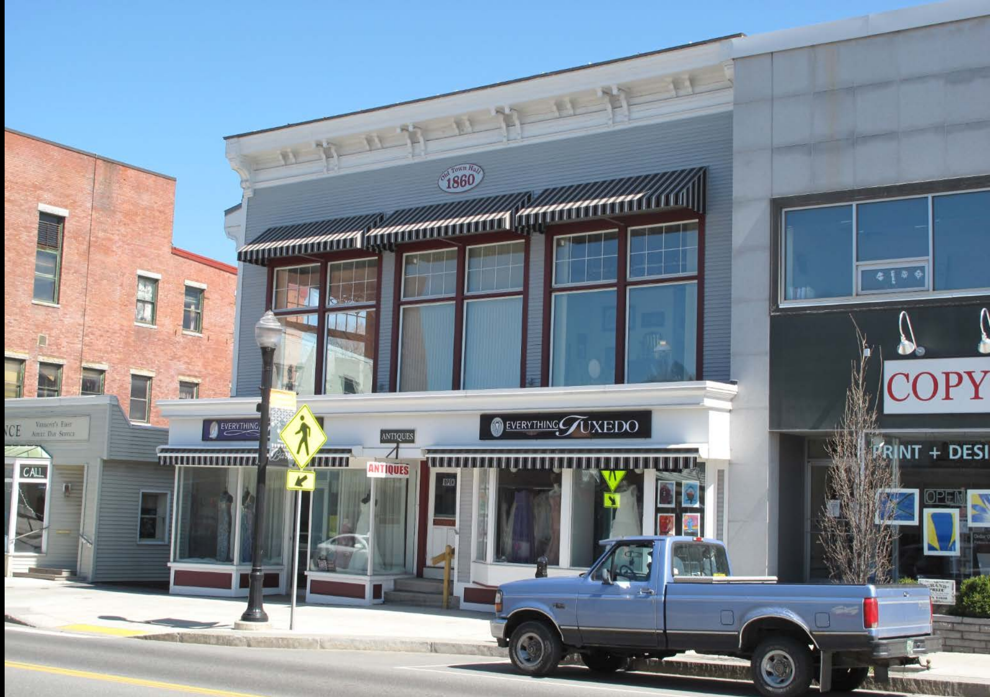
Photograph 59: View looking north at Commercial Building (left), HD #45, and Old Town Hall (center), HD #46
