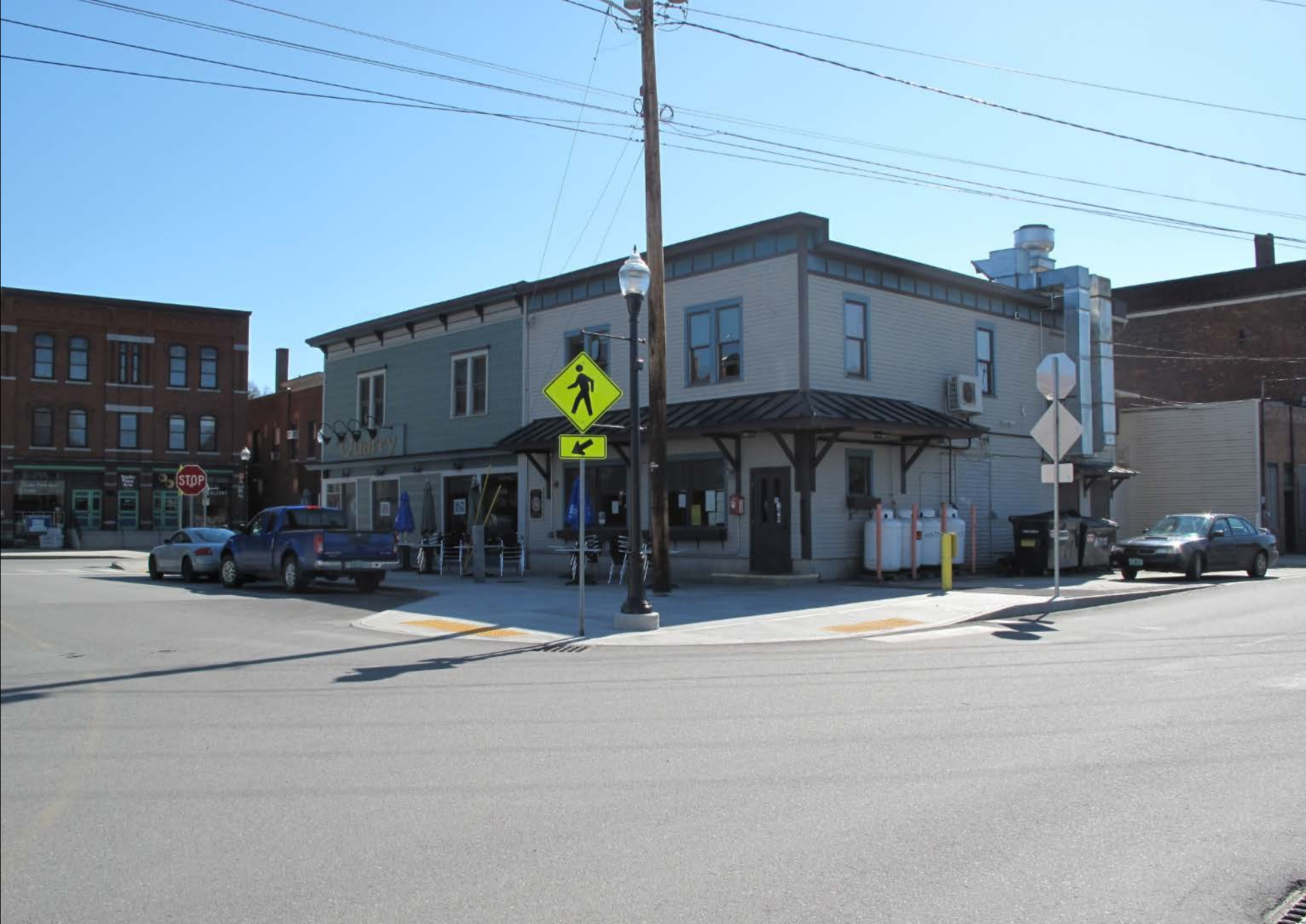
Photograph 48: View looking east at Commercial Building (left), HD #33, and Commercial Building (center), HD #34
