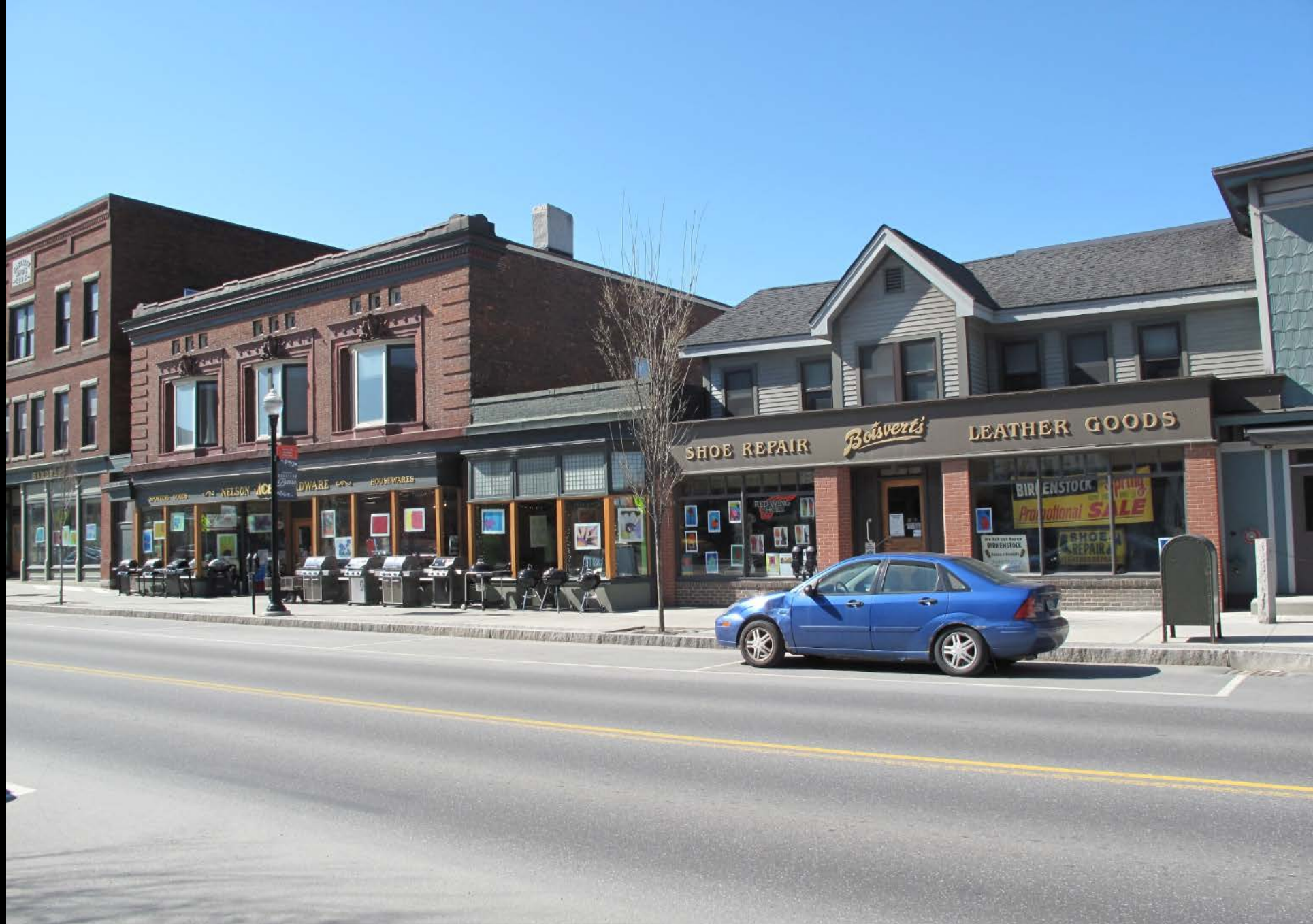
Photograph 46: View looking southwest at Commercial Block (far left), HD #31,
