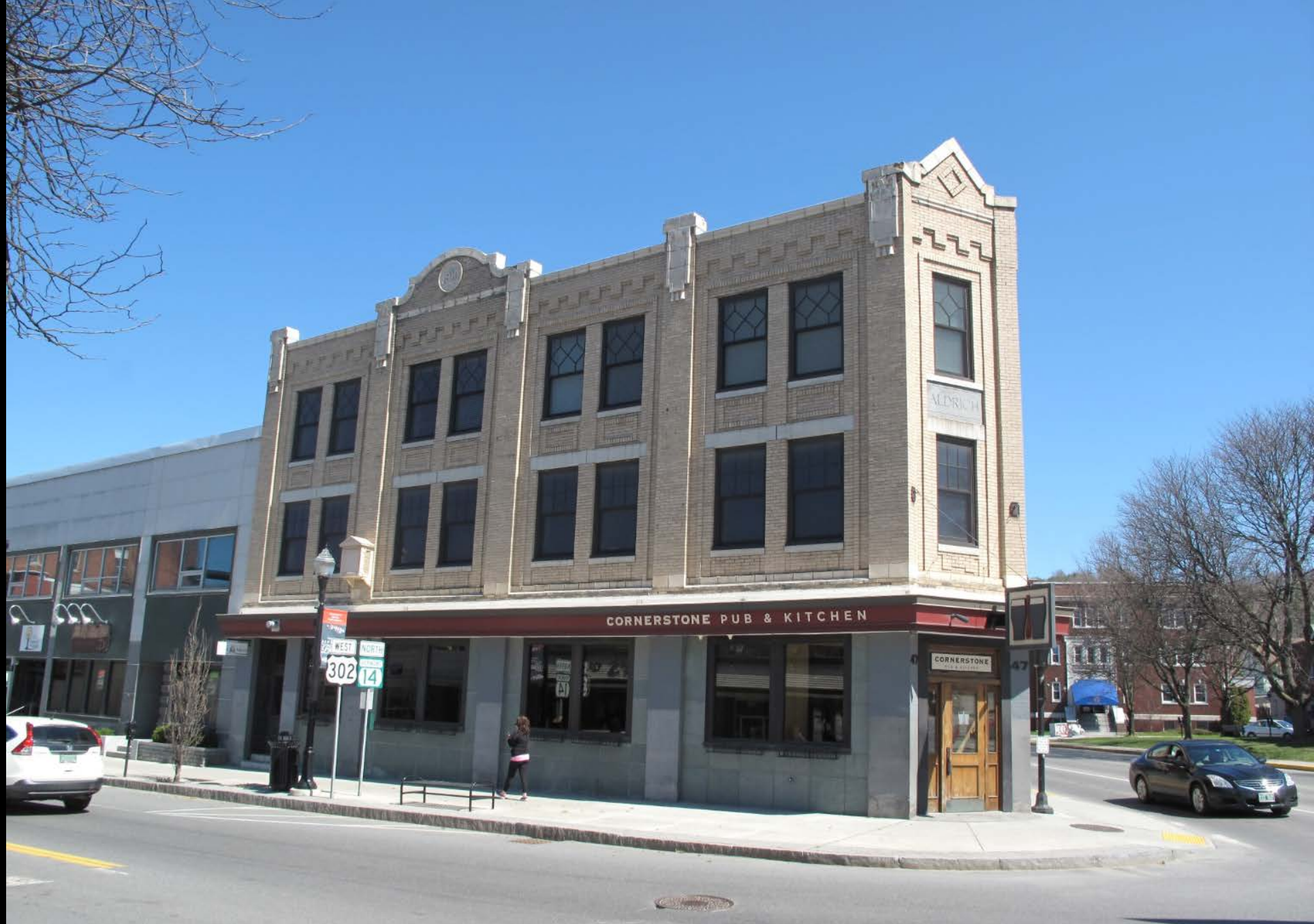
Photograph 61: View looking north at Aldrich Block, HD #48
