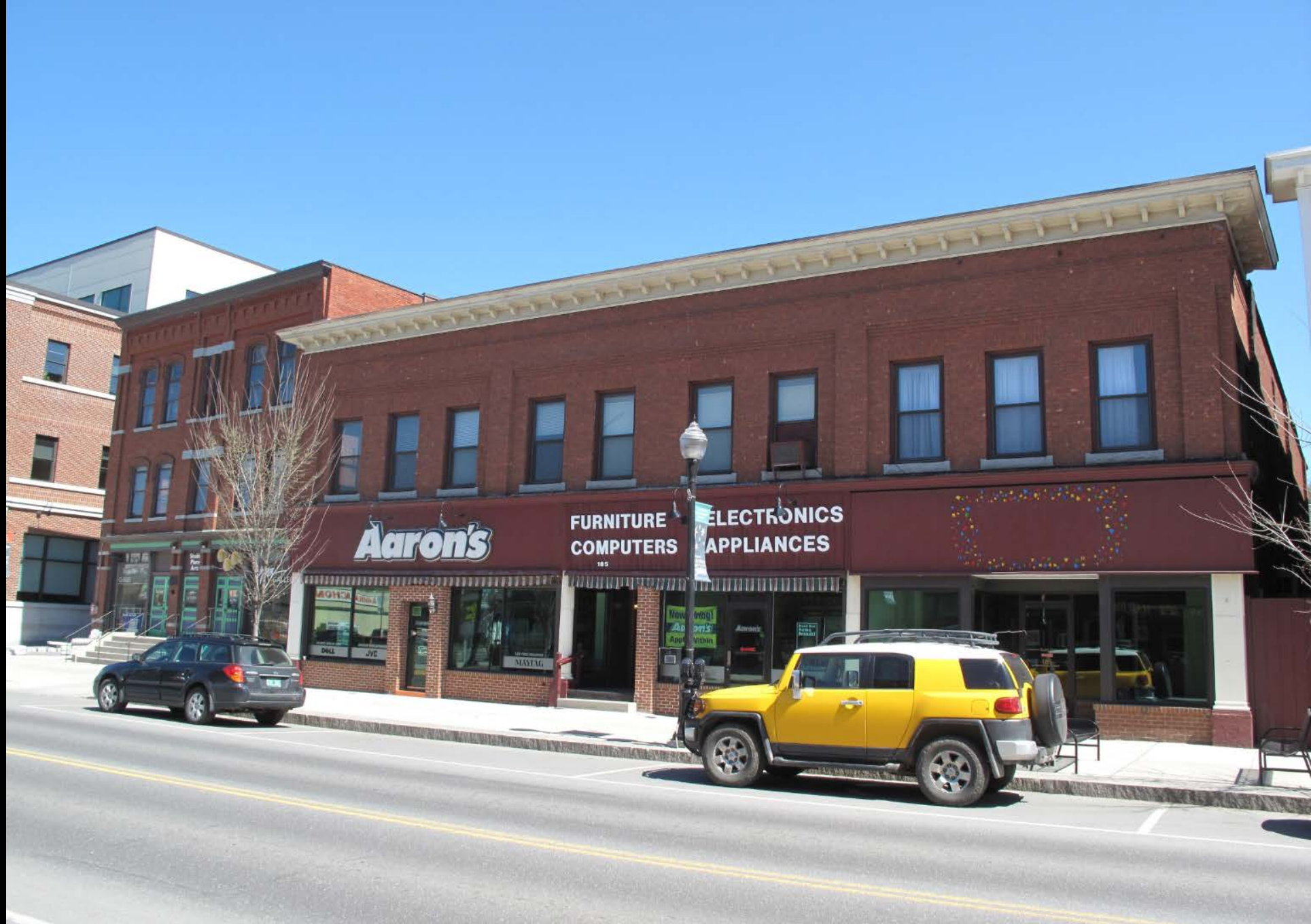
Photograph 52: View looking north at Currier Block, HD #37
