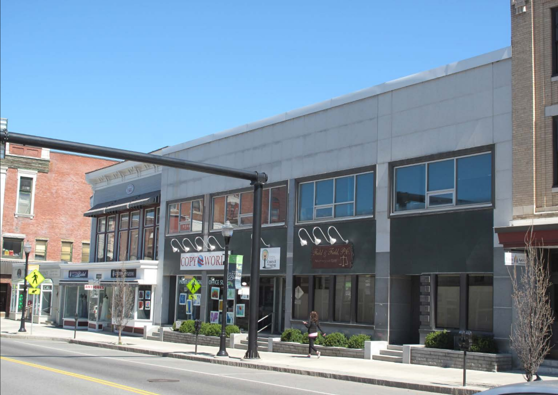
Photograph 60: View looking north at Stillman Wood Block, HD #47
