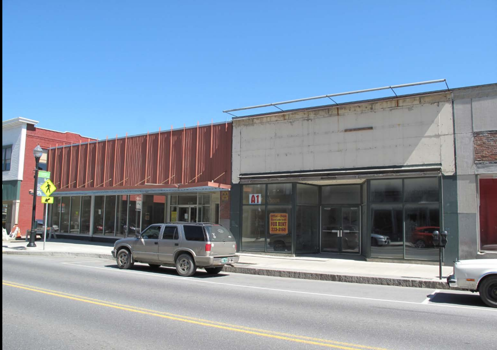
Photograph 55: View looking north at Commercial Building, HD #40
