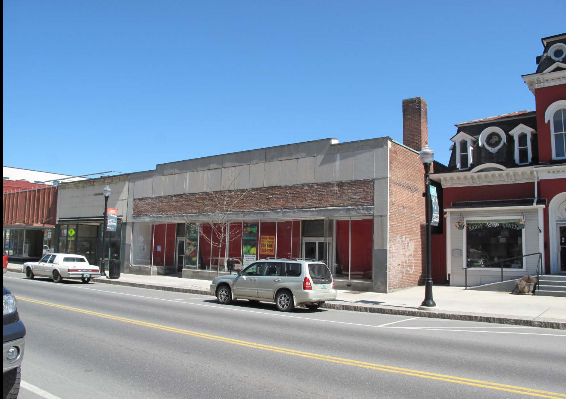
Photograph 56: View looking north at Commercial Building, HD #41
